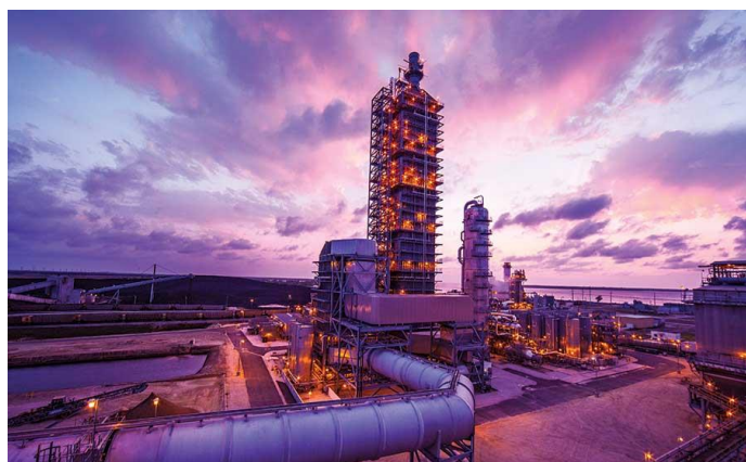
Figure 1. Petra Nova, located near Houston, TX, utilizes a post-combustion capture system and then transports the captured carbon via pipeline to an oil field for enhanced oil recovery. Source: NRG.
