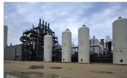
Air Products Port Arthur, TX Hydrogen Production Facility
